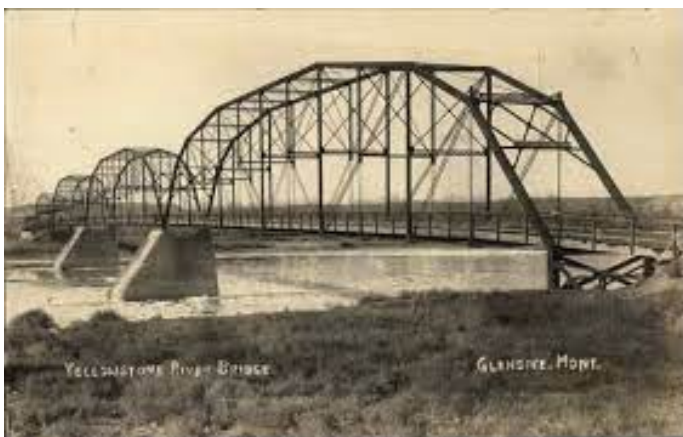
Yellowstone River Bridge, Glendive Montana
