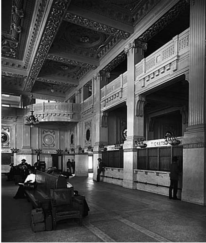
Seattle's King Street Railroad Station
